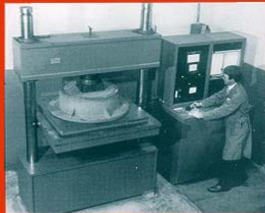
To determine load bearing qualities of Neenah castings, press tests are conducted as part of our research program. Write for our wheel load capacities manual.
