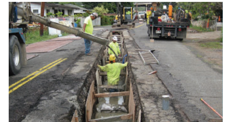
Construction of local sewer by open cut (trench)
